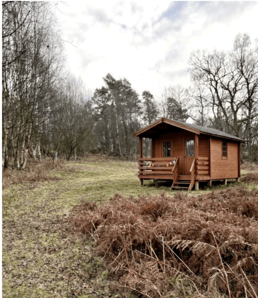
An artistic impression of a new retreat hut on Site 1: Please note: the design differs slightly to what will be constructed
